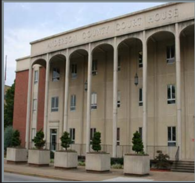
Anderson County Courthouse
