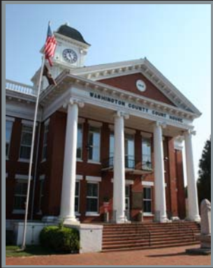
Washington County Courthouse
